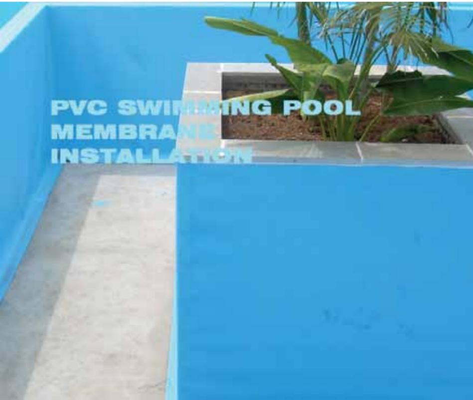
The 1.5mm (60mil) PVC Pool Shell Lining systems for Swimming Pool Renovations and New Pool Construction projects are available in solid and printed color designs, the vinyl liner waterproof membrane material will beautify and protect any new or existing project.
