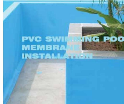
Next, the second layer of adhesive is installed to both the fleece padding and the PVC waterproof membrane at all vertical walls including the deep end walls. All lap seams are thermoplastic welded and a special chemical seam sealer is applied to the seams edge for added protection. The waterproof PVC shell can be installed with or without lane markers, custom logos and a special non skid surface material can be installed at stairs, ramps, in shallow water pools or splash pads
